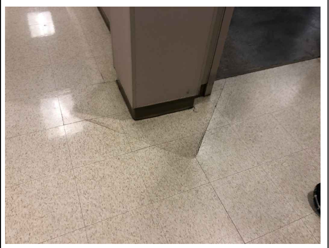
② EXISTING CONDITION AT 28 FLOOR DEPRESSION
