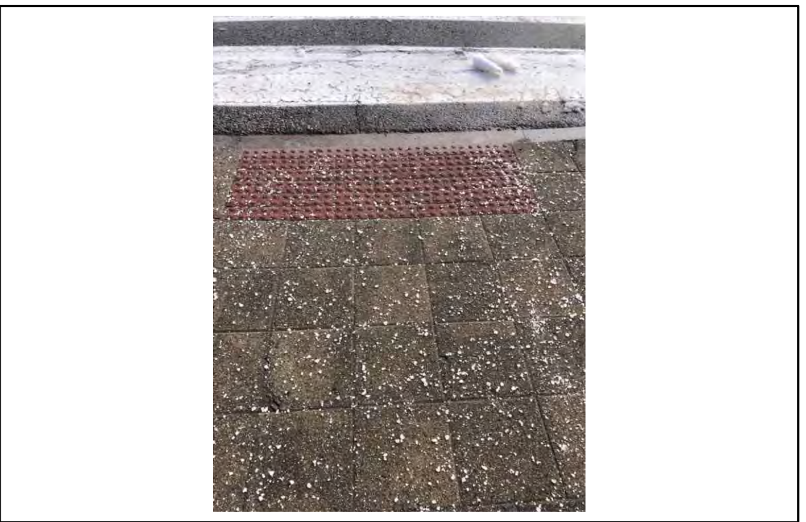
② EXISTING DETECTABLE WARNING STRIP - FOR REFERENCE ONLY
