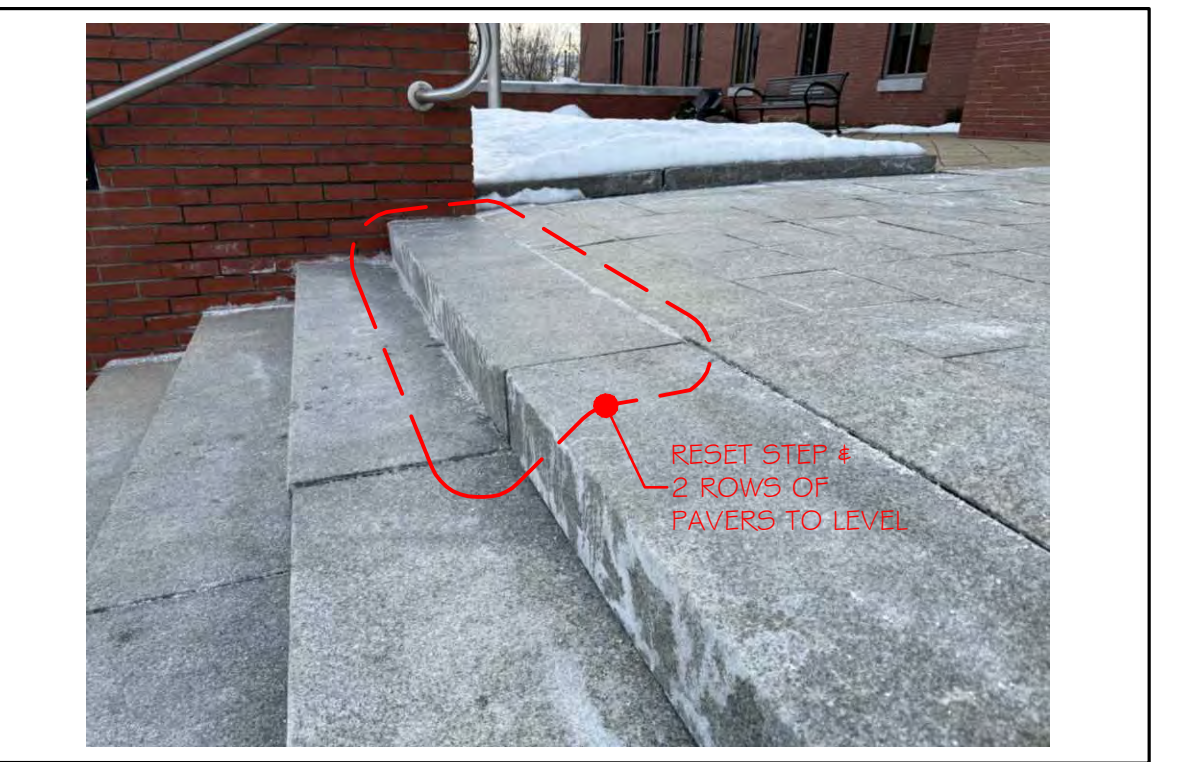
③ RESET EXISTING GRANITE STEP/PAVERS
