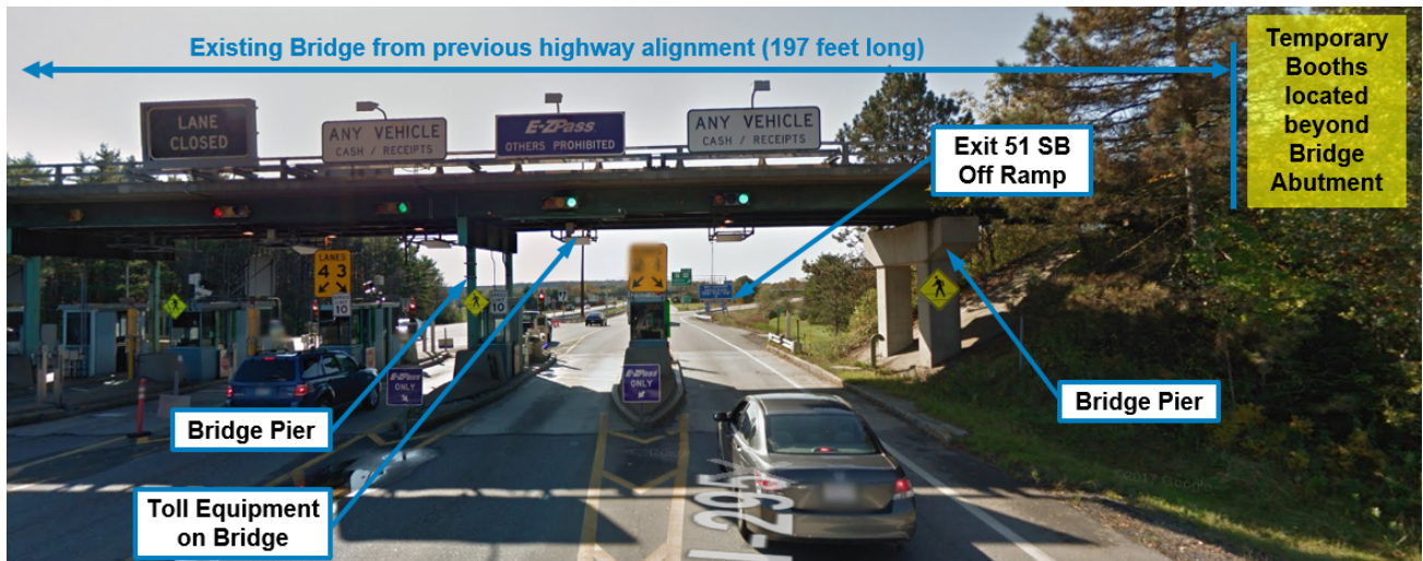
Figure 3 – Southbound View of Existing Plaza
