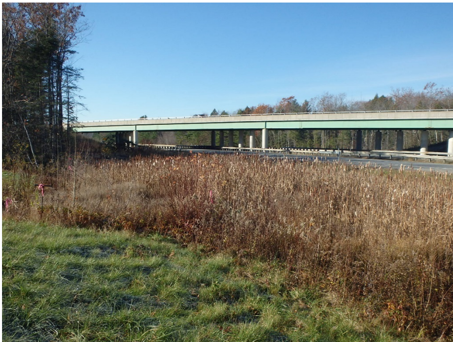
Photo 4. Wetland D: Typical PEM wetland along I-95 off-ramp to I-295 southbound; impounded by roadway and culvert outlets to Wetland C. Stantec, November 9, 2017.
