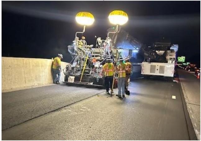
Coastal Road Repair's paving crew finishing up the median shoulder paving against the concrete barrier.
