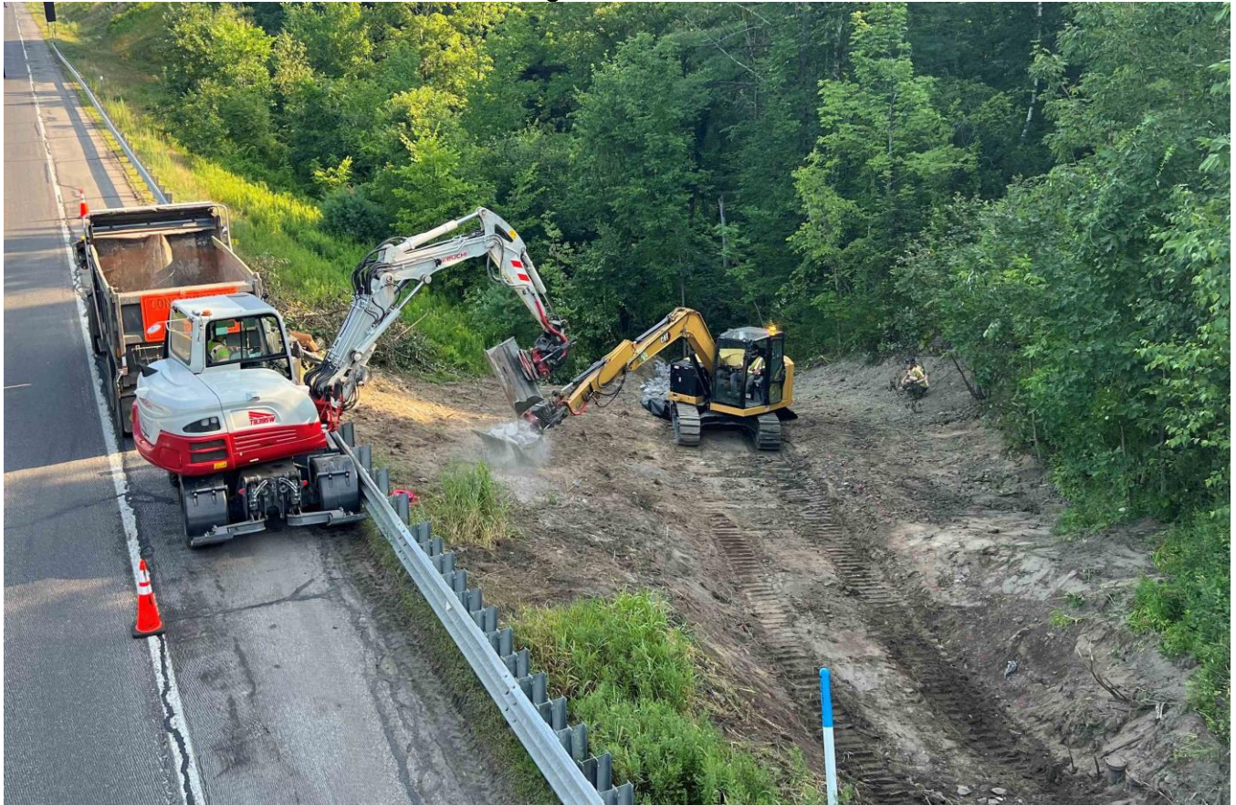
Taken from Mountain Road in Falmouth, crews work to repair a ditch washout.
