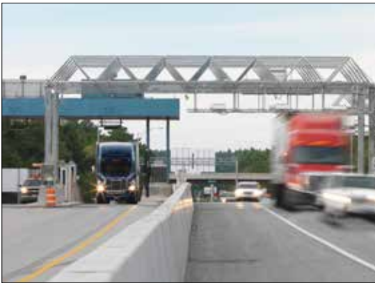
NEW GLOUCESTER TOLL PLAZA
