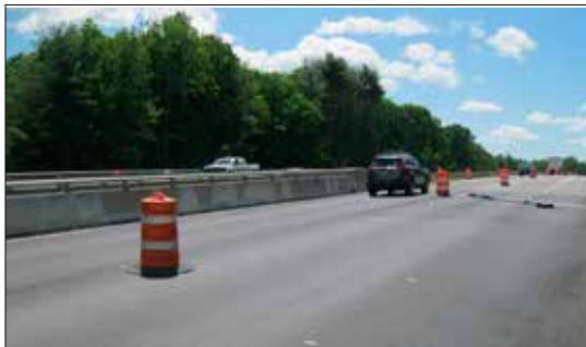
HUNTS HILL ROAD OVERPASS, MILE 61.6
