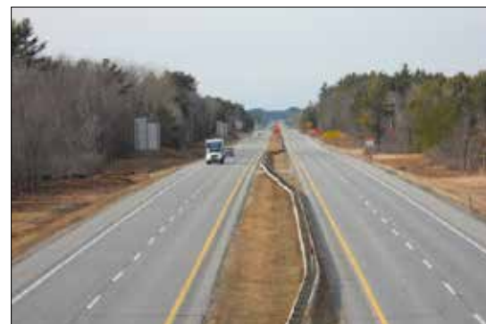
ROADWAY SIDE SLOPE CLEARING LOOKING SOUTH, MILE 102 (AFTER)
