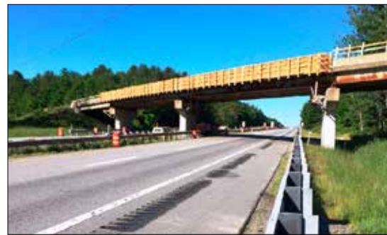
SMALL ROAD UNDERPASS, MILE 95.1
