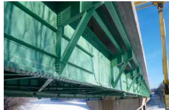
ANDROSCOGGIN RIVER BRIDGE
