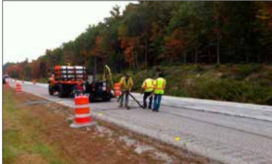
DISPENSED AT OVER 350 DEGREES THE RUBBERIZED ASPHALT SEALANT IS INJECTED DIRECTLY INTO THE PAVEMENT CRACKS
