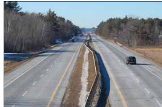
ROADWAY SIDE SLOPE CLEARING LOOKING SOUTH, MILE 102 (BEFORE)
