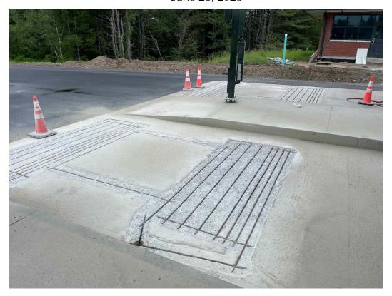
The Exit 35 Southbound Lanes 1 and 2 grooves cut prior to loop installation.
