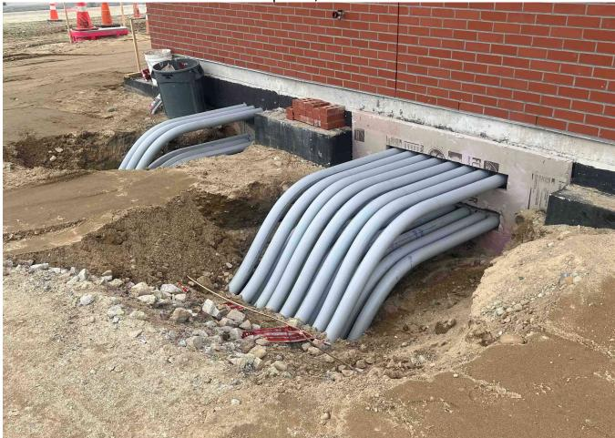
A bank of conduits for electrical and communication lines from the toll plaza to the admin building are prepped for backfilling with sand.
