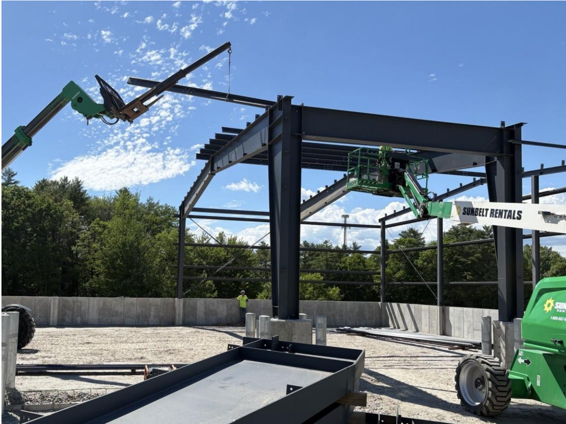
The Pre-Engineered Metal Building installation is in progress.
