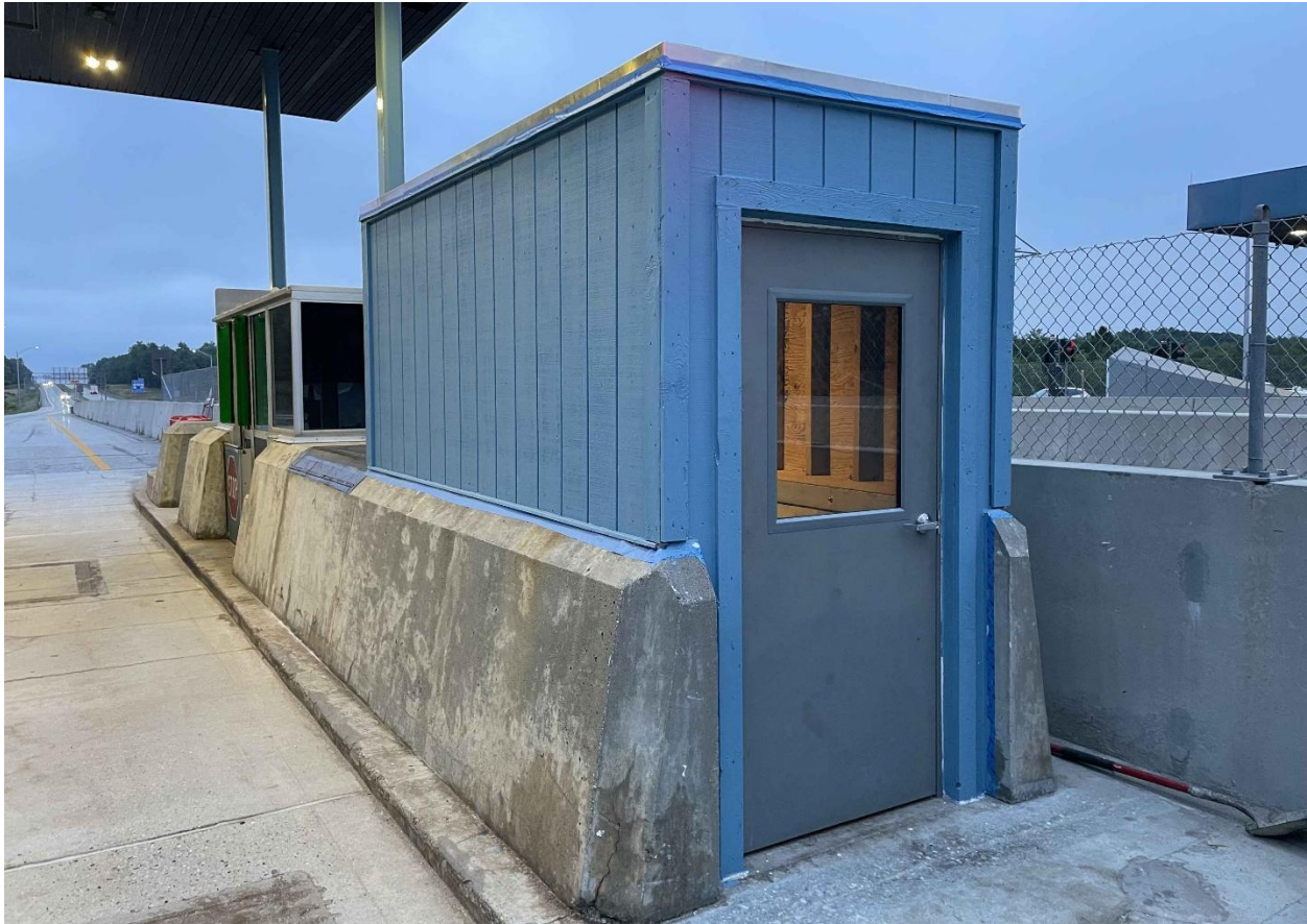
Looking at West Gardiner Toll Plaza southbound stair enclosure for tunnel access.
