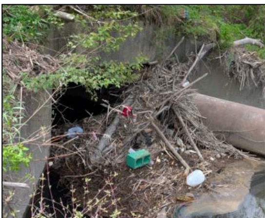
Image 1 – Debris at Culvert Inlet
