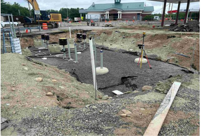
The new fuel tanks are buried under the crushed stone with various connections being installed into the tank system.
