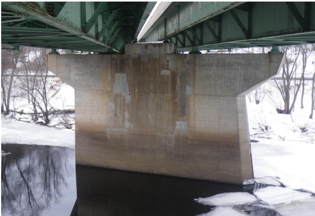
**Figure 2 View of Pier Concrete Deficiencies.**
