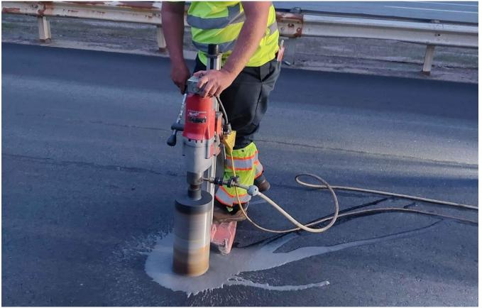
Pike's quality control technician is cutting a core to check for pavement density.
