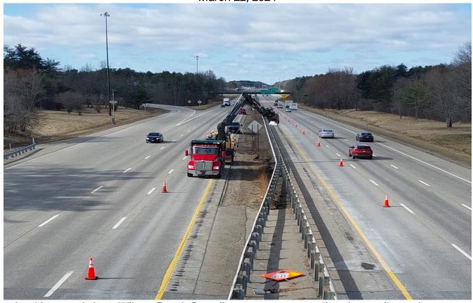
Looking south from Wilson Road, Grondin crews are re-grading the median to improve drainage
