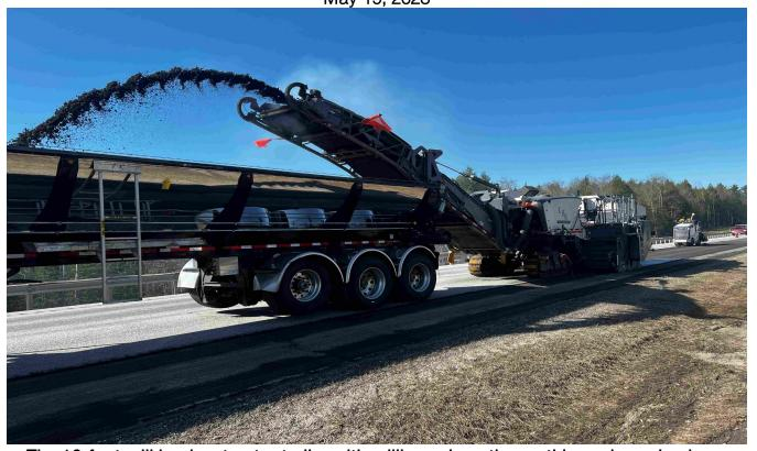
The 12-foot mill loads a tractor trailer with millings along the northbound passing lane.
