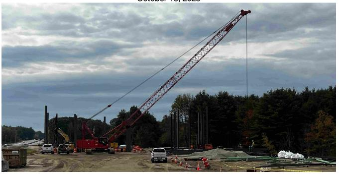
Looking at the new southbound plaza, a crane is lifting and setting piles for the toll structure.
