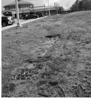
ANSWER: Likely captures 10% of flows. The lack of vegetation will generate erosion and sedimentation as seen with the channelized flow. No vegetation to dissipate flows and buffer pollutant loads. Covered CB is likely clogged internally also.
