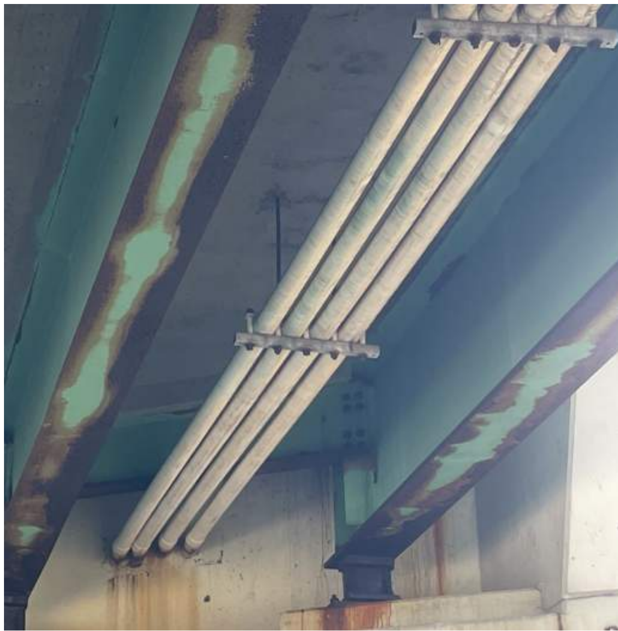
Photo: Utility conduits in southernmost girder bay
