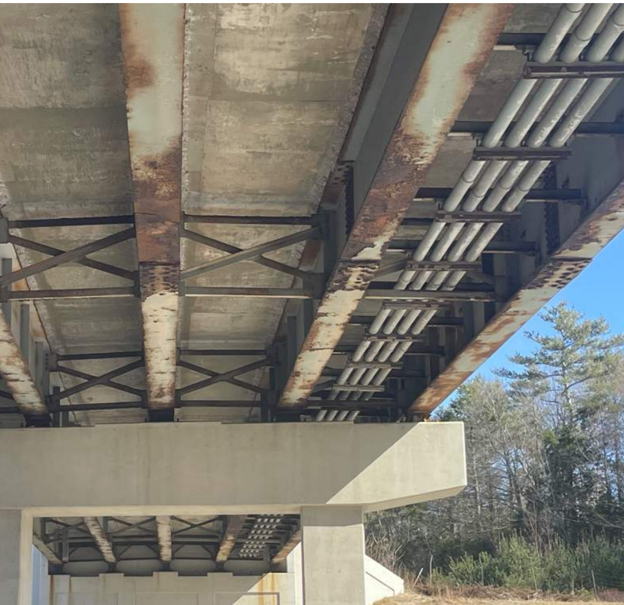
Photo: Utility conduits in southernmost girder bay
