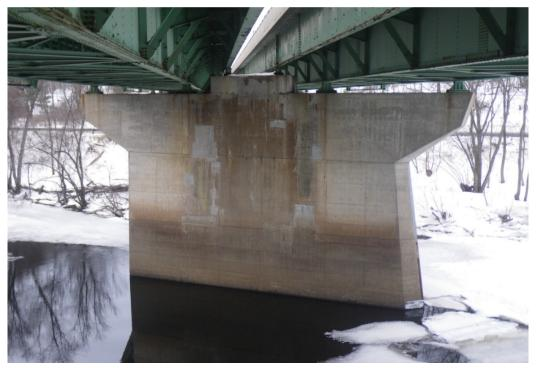
Figure 2 View of Pier Concrete Deficiencies.
