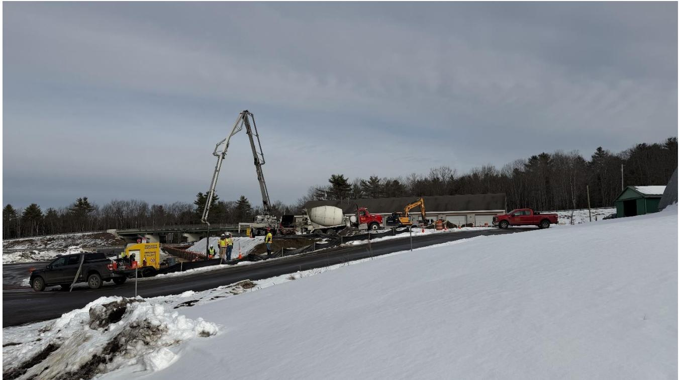
The contractor places the foundation footing along the back wall of the new Vehicle Storage Garage
