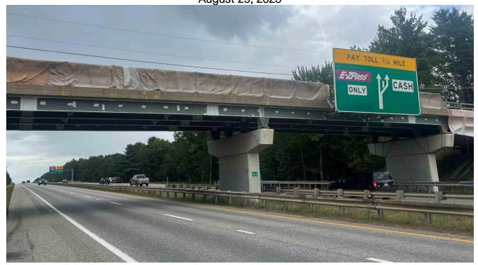
Saffo Contracting has mobilized containment and access equipment to Shaker Road Bridge where they will be replacing the paint system.
