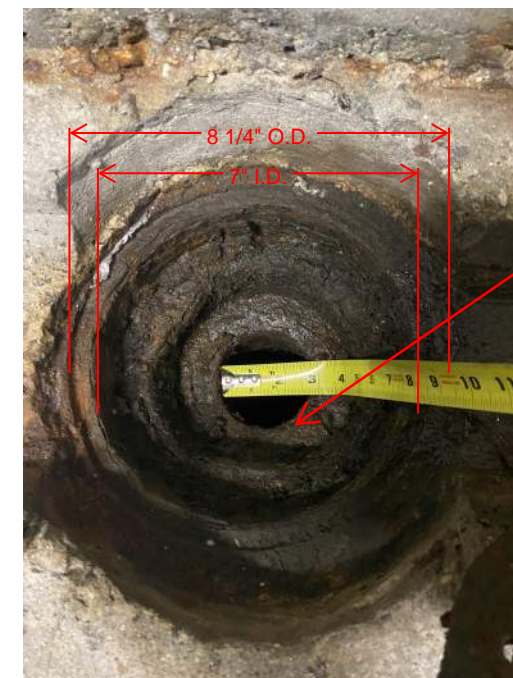
EXISTING FLOOR DRAIN DETAIL
