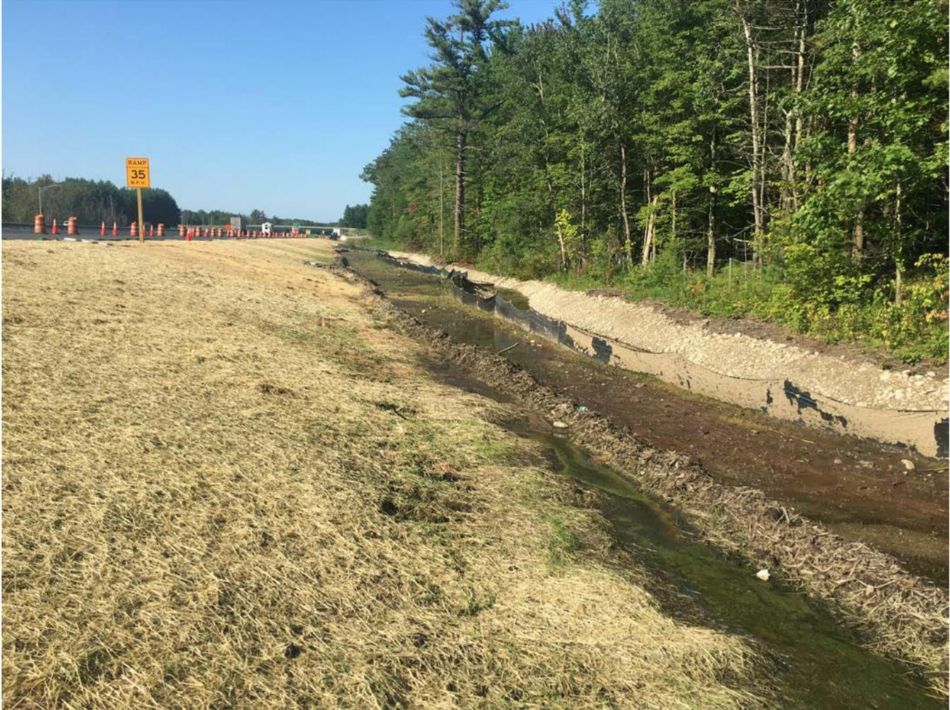
**Photograph 1 – August 2021 photograph of relocated stream and re-constructed riparian wetlands along an unnamed tributary to Thatcher Brook within the UA boundary in Biddeford at Exit 32 southbound.**
