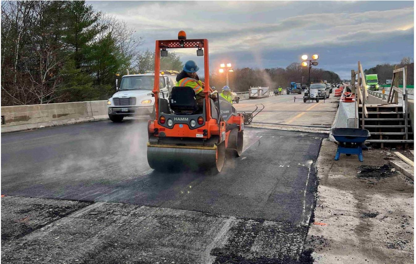
A roller compacts an intermediate layer of pavement at the north end of the northbound Androscoggin River bridge
