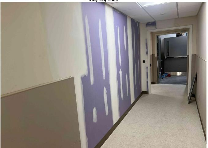
One of the walls that were repaired as part of the boiler stack replacement on the first floor
