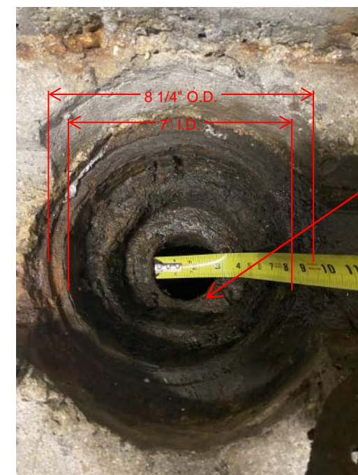
EXISTING FLOOR DRAIN DETAIL
