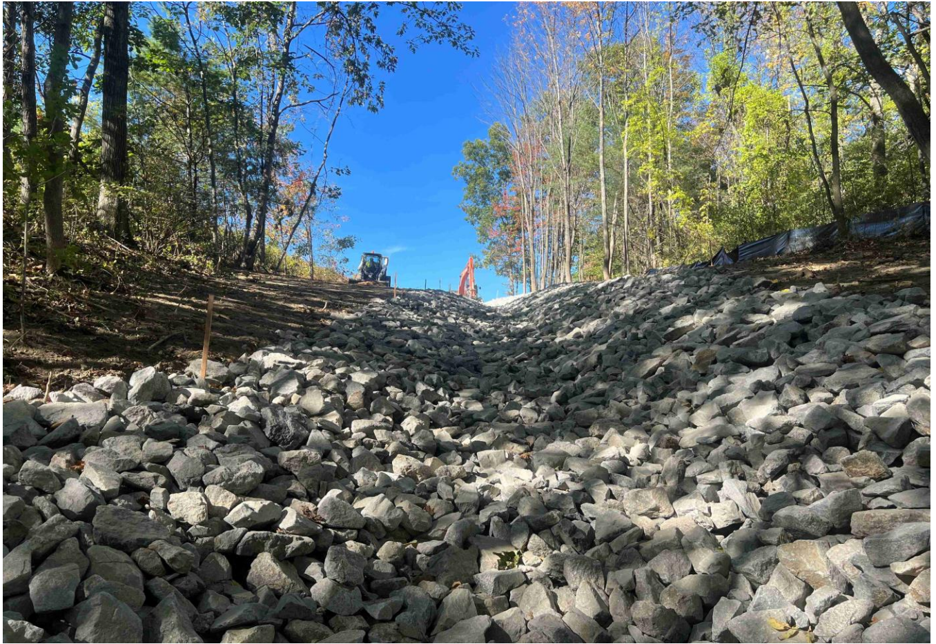
Mile 57 northbound in Cumberland, a new ditch was built to replace a failing pipe
