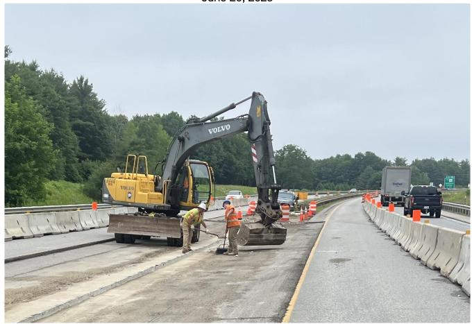
Laborers and an excavator are cleaning up around the median drainage prior to paving the crossovers. They will be needed when the bridge joints are replaced.
