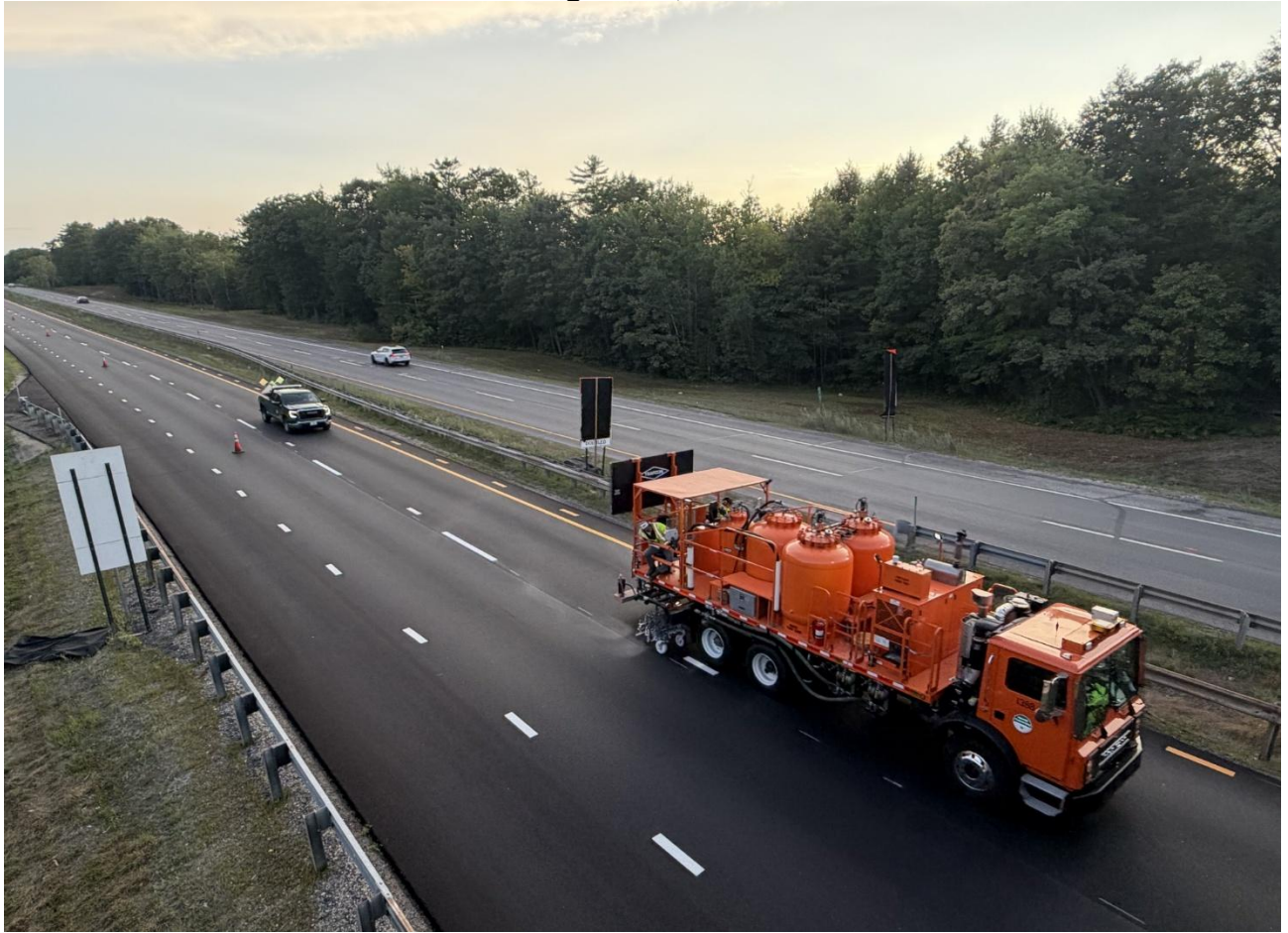
The MTA paint truck applies final striping on the northbound lanes in Gray.
