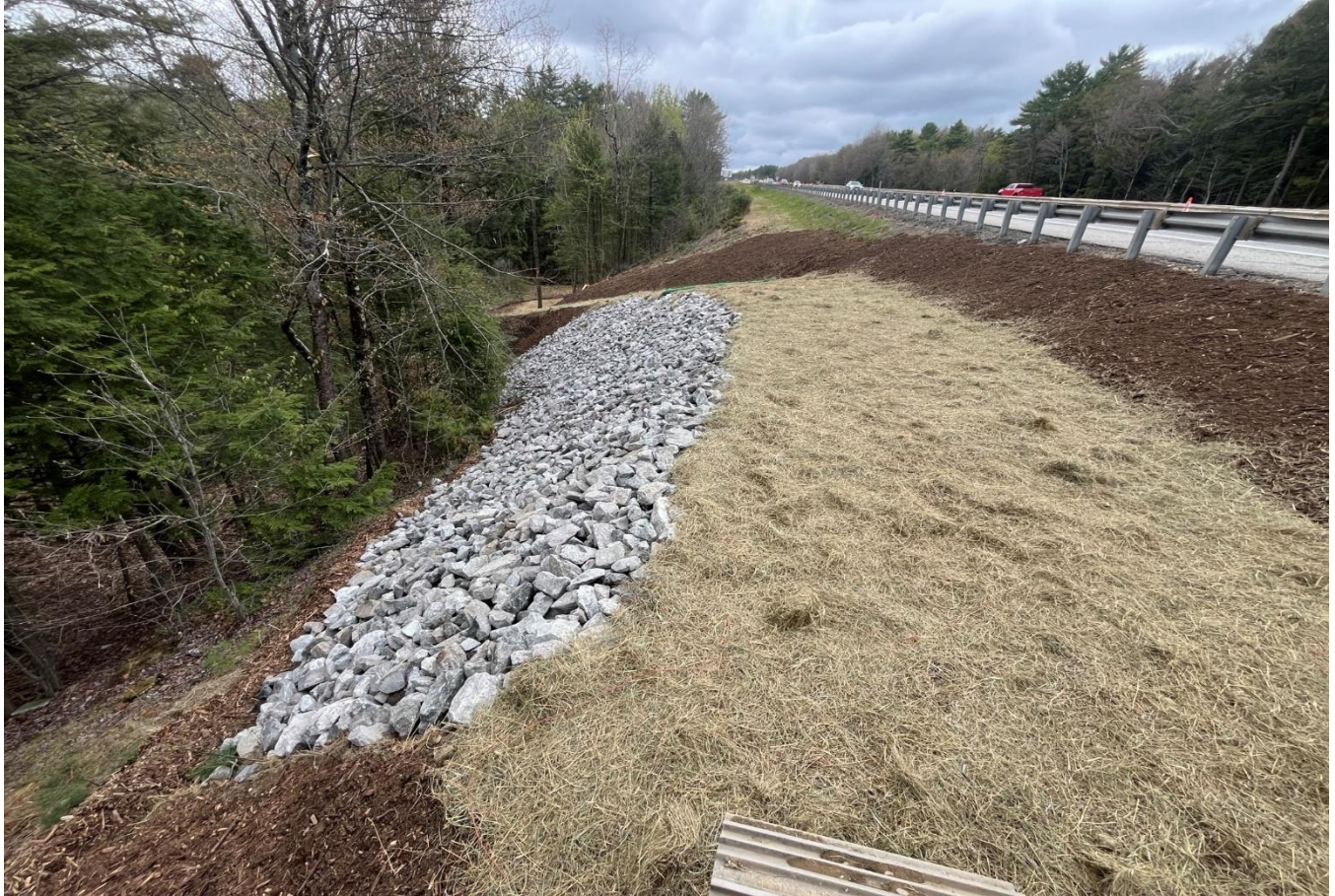
Access to outlet end of Mile 72.0 culvert (Northbound)
