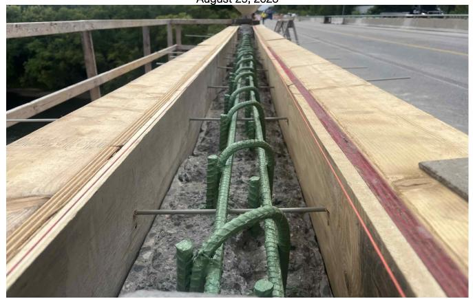
Looking south at the concrete barrier with forms and reinforcing steel all prepped for new concrete.
