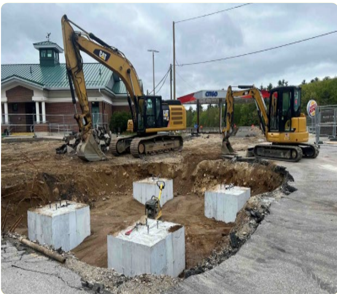
Photo 14: Cumberland Service Plaza Construction
