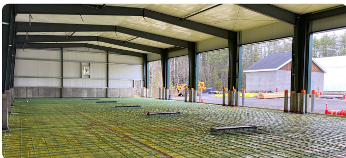
Photo 17: York Maintenance Eight-Bay Garage Construction
