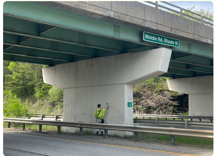
Photo 19: Median Pier Inspection
