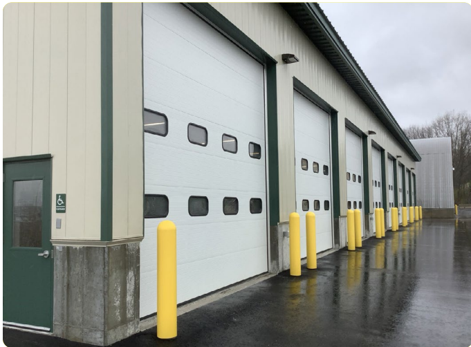
Photo 16: Crosby Maintenance Eight-Bay Garage
