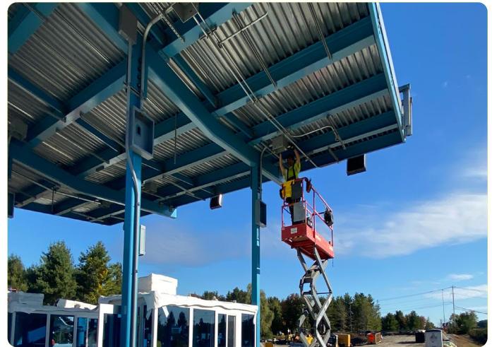
Photo 13: Saco Toll Canopy Construction
