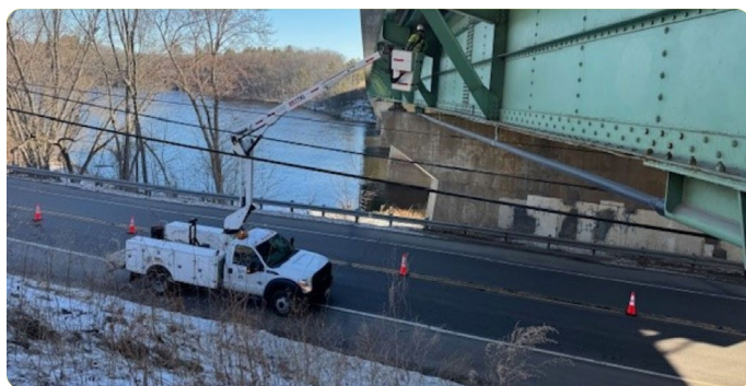
Photo 20: Androscoggin River Bridge Inspection
