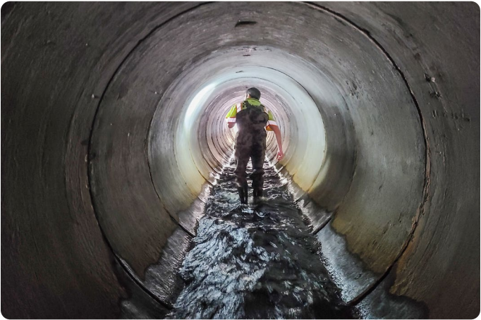
Photo 3: Large Diameter Culvert Inspection
