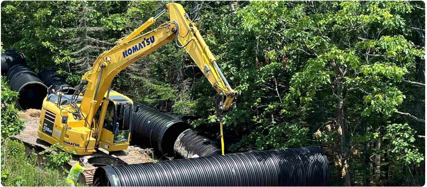
Photo 5: Culvert Slip Lining
