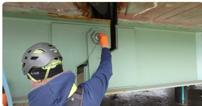
Photo 21: York River Bridge Pin-and-Link Inspection
