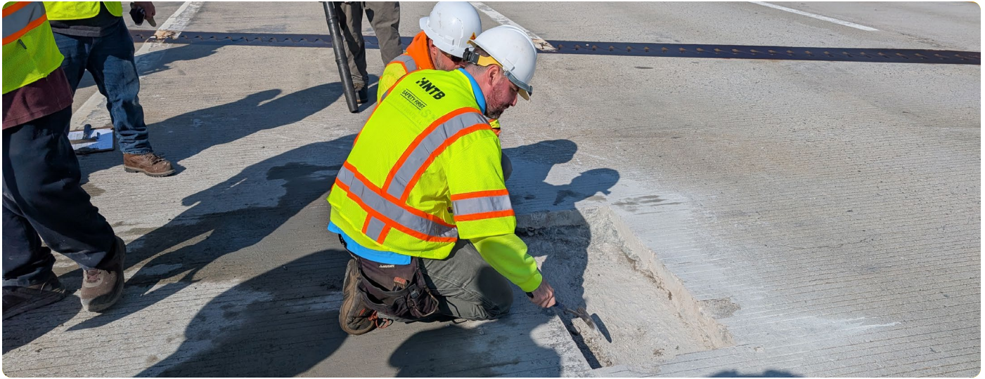
Photo 26: York River Bridges Wearing Surface Repair
