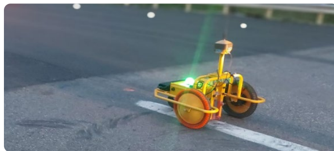
Photo 9: Robotic Striping Layout (Operated by Pike Industries)
