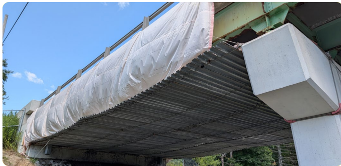
Photo 24: Bridge Painting Containment System
