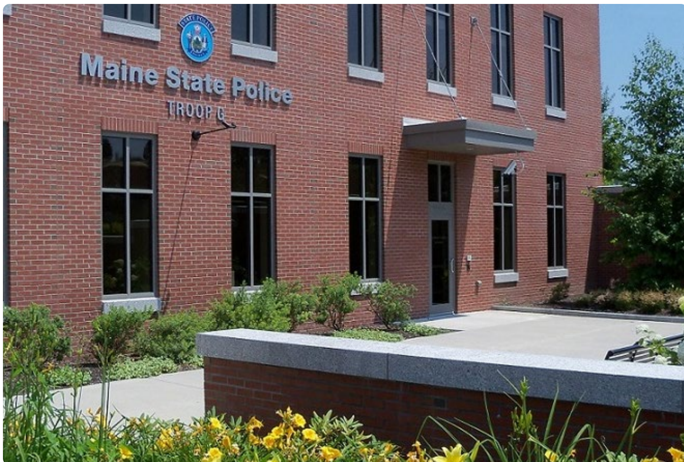
Photo 29: MTA Administration Building Maine State Police Troop G Entrance
