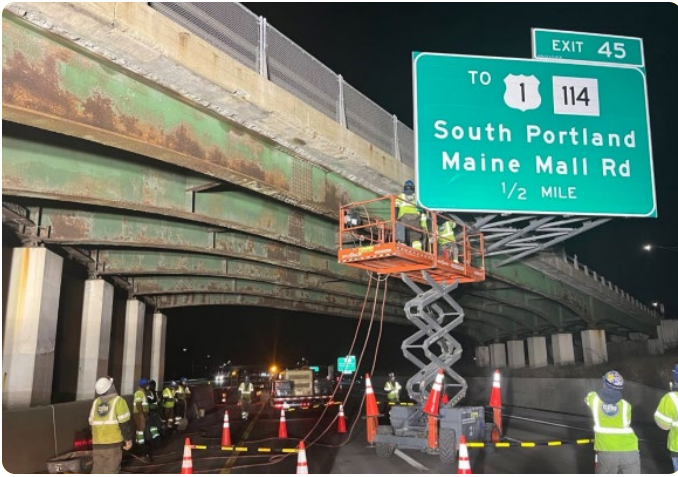
Photo 25: I-295 SB Underpass Haunch Removal
