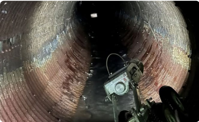
Photo 4: Vortex Small Diameter Culvert Inspection (Not an MTA Culvert)
