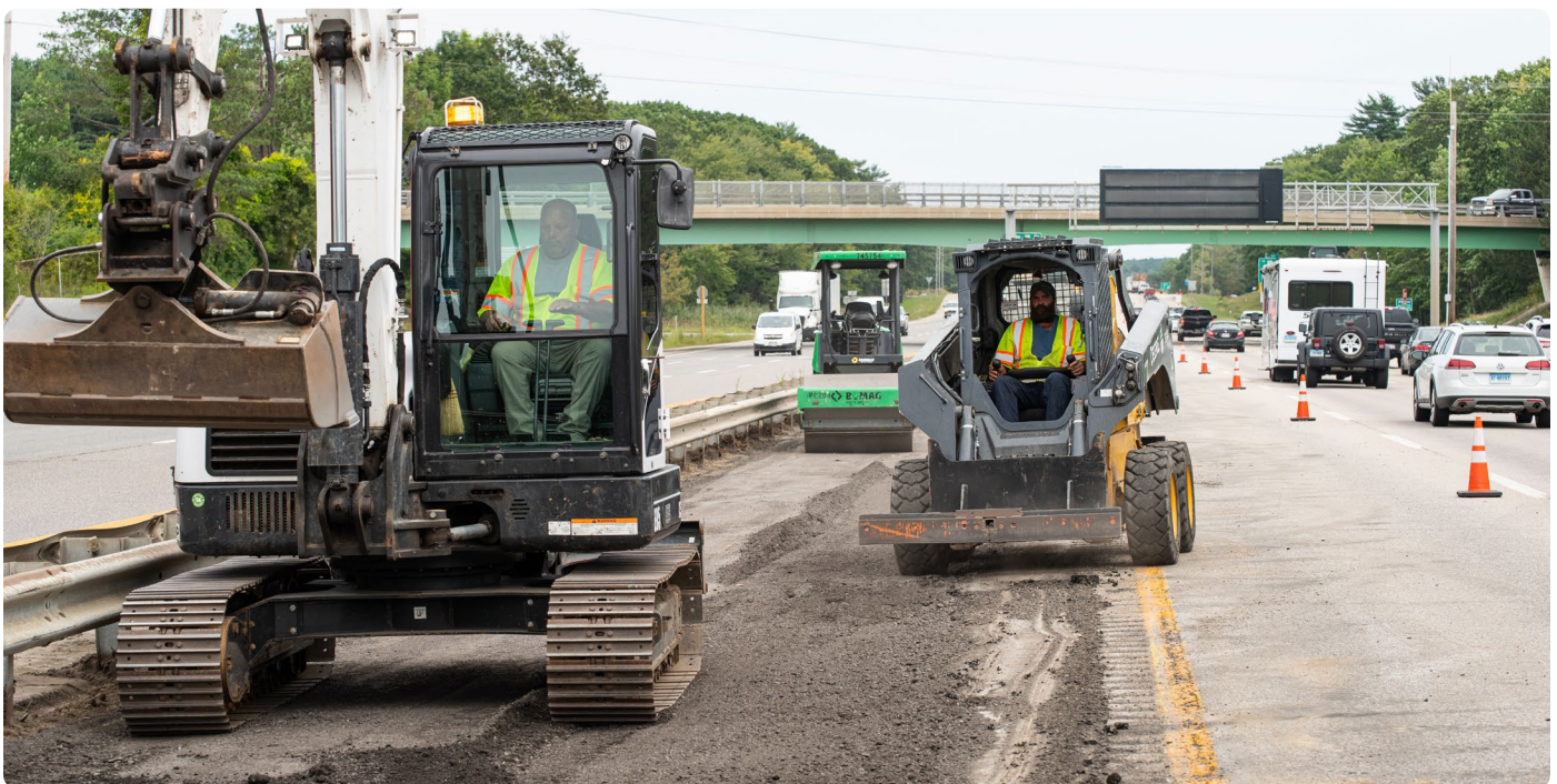
Photo 10: Median Grading Operations
