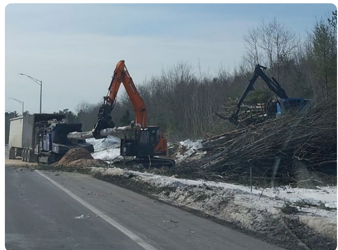
Photo 8: Roadside Clearing Operations
