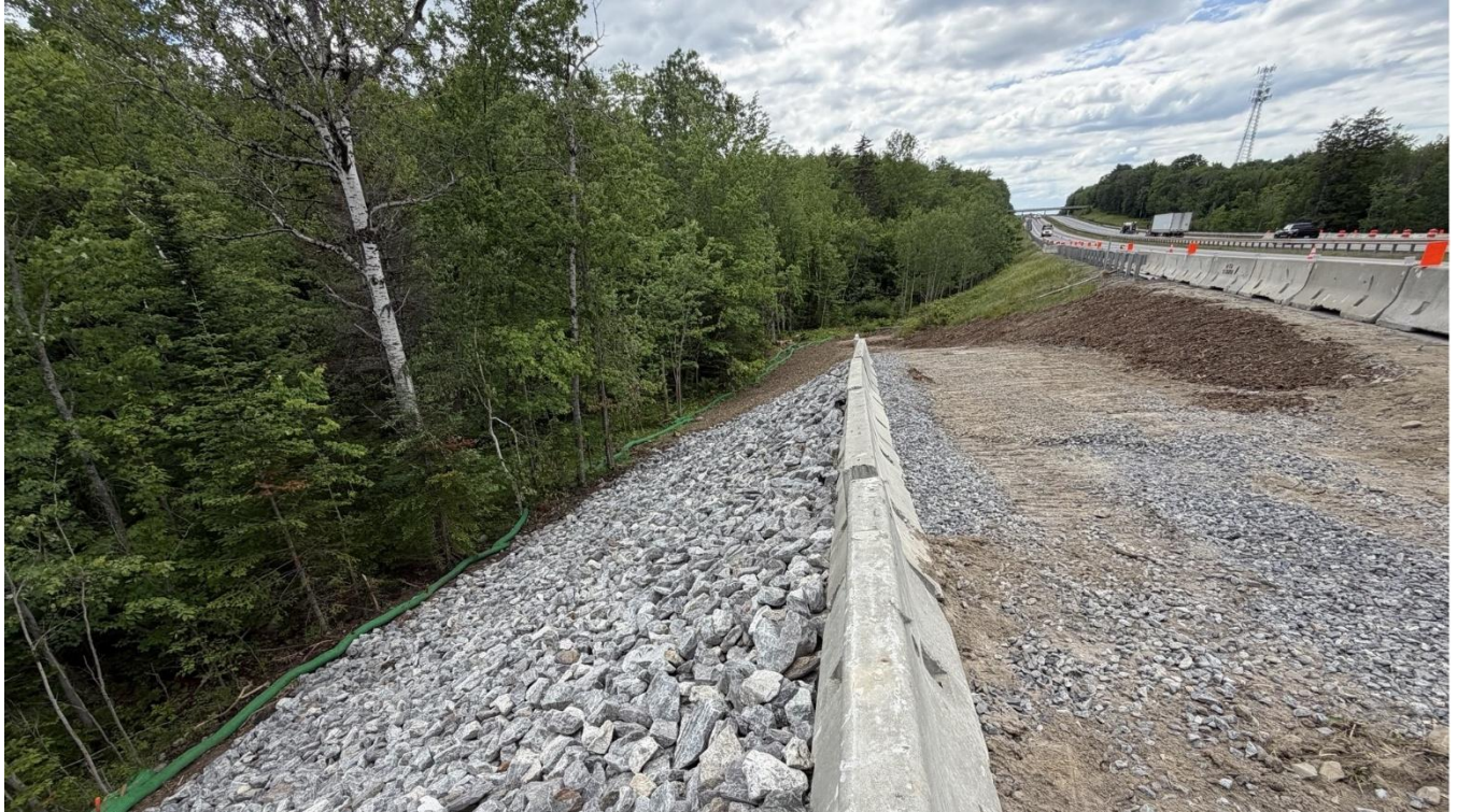
Access to outlet end of Mile 91.3 culvert (Northbound)
