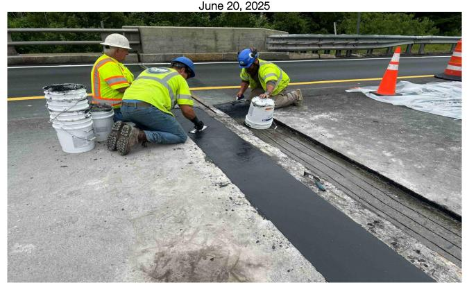
The contractor performs an elastomeric concrete header replacement on northbound lane 1
