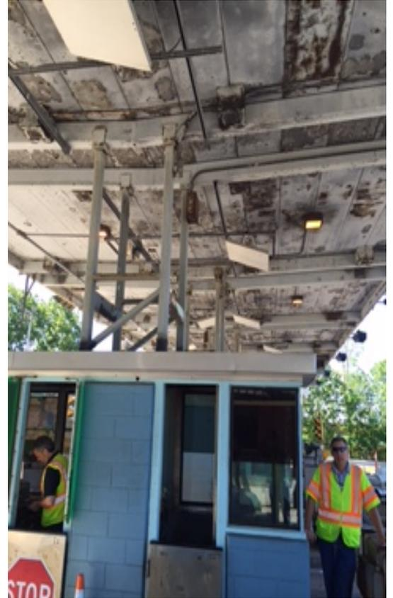
**Figure 2: Roof Support beams lead paints**
