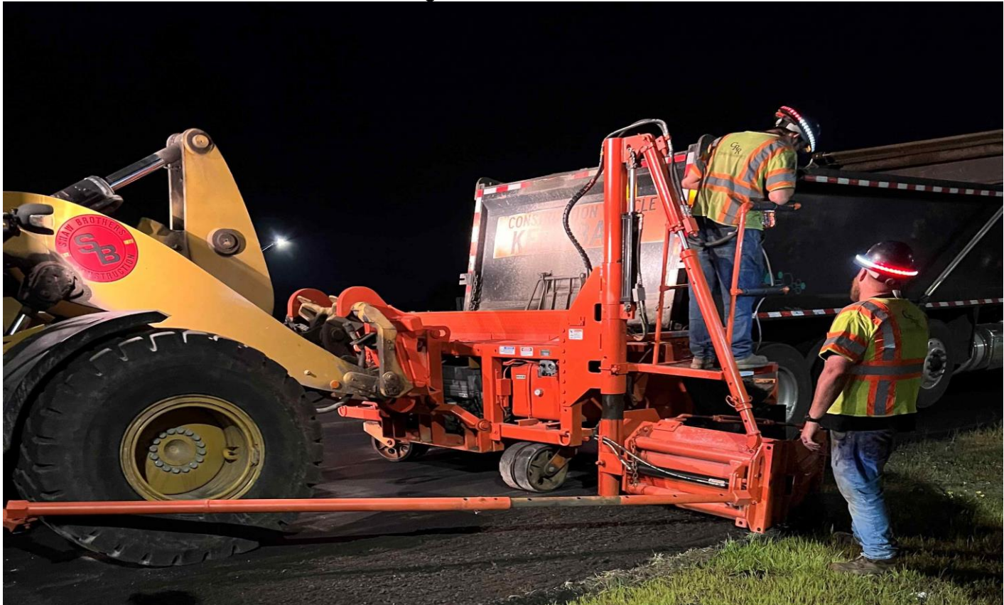
Coastal Road Repair operating a shoulder machine backing up the new pavement.
