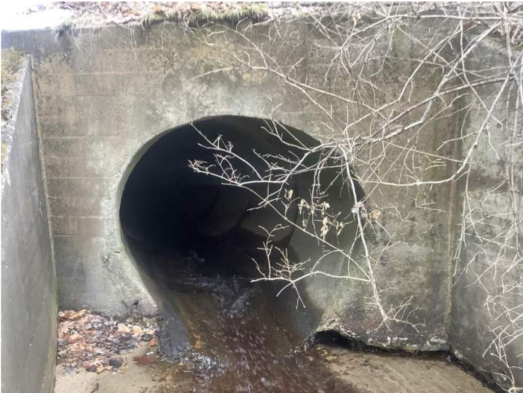
Photo #6: Headwall Scour at Culvert Outlet.
