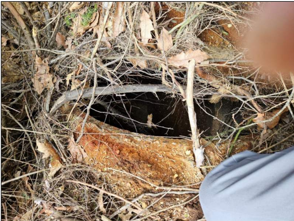
Photo #8: Joint Separation in Culvert Pipe Before Repair. (Photo from HNTB 2024 Damage Assessment and Recommendation Report)
