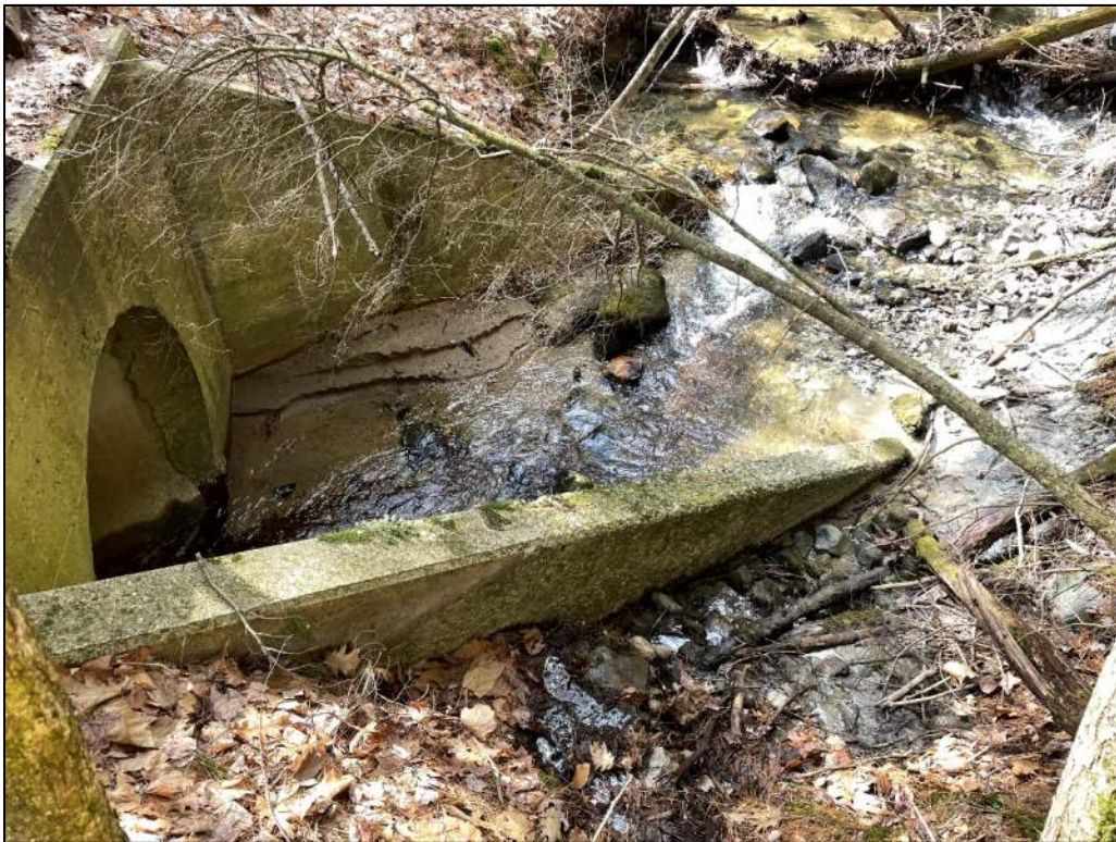
Photo #2: Culvert Inlet.
