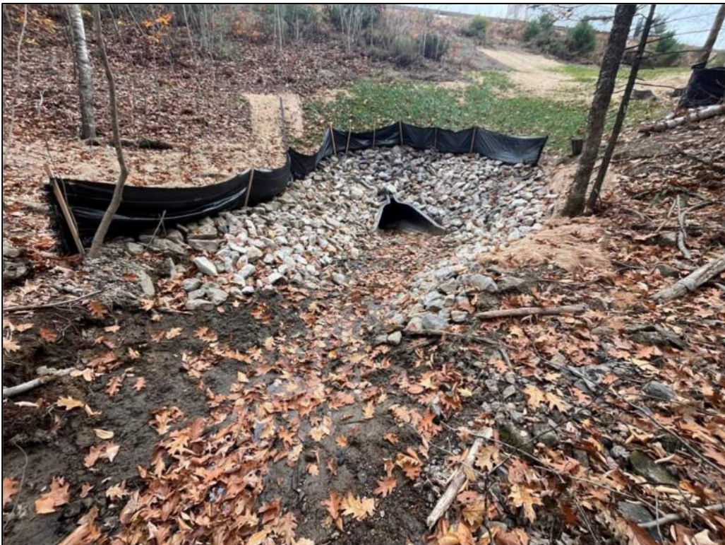
Photo #2: Culvert Inlet. (Photo from MTA 2024 Slope Culvert Repair Report)
