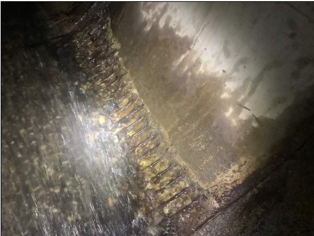
Photo #8: Heavy Spalling with Exposed Rebar Under Southbound Barrel. (Photo from MTA 2022 Annual Inspection Report)
