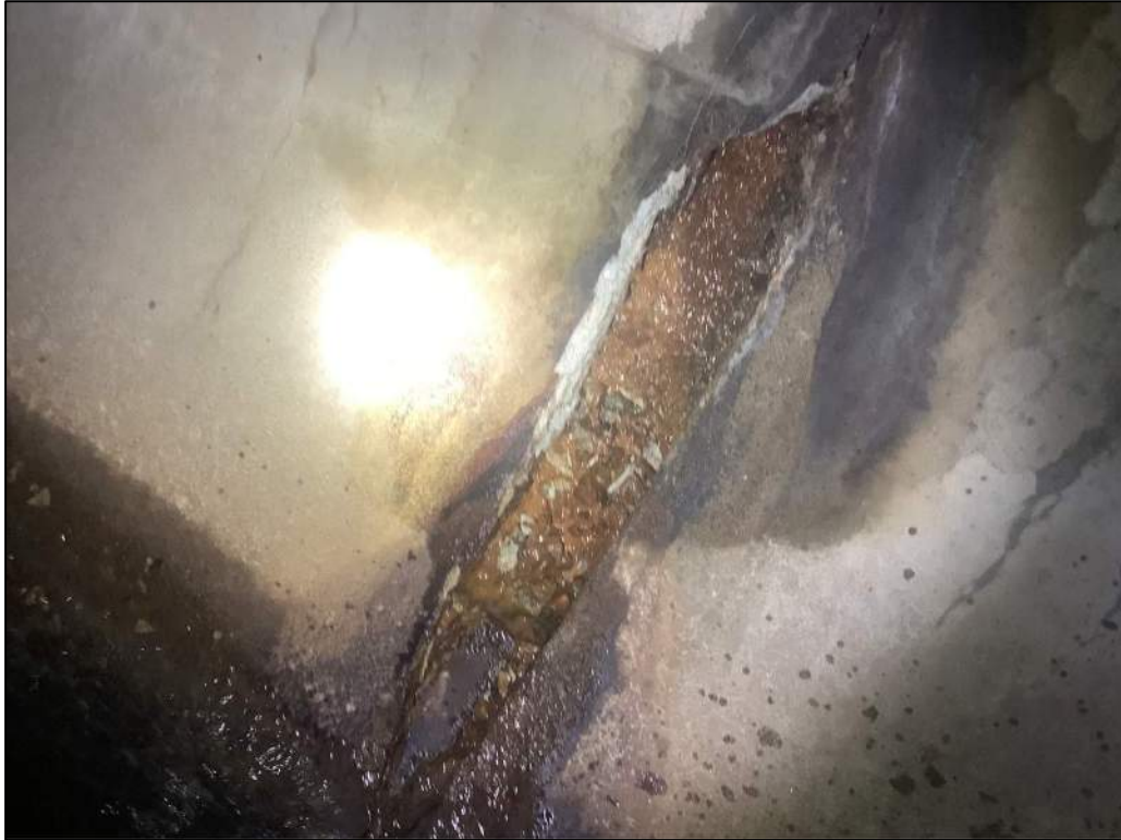
Photo #7: Culvert Joint Deterioration Under Northbound Barrel. (Photo from MTA 2022 Annual Inspection Report)
