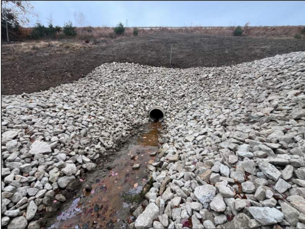
Photo #5: Culvert Outlet. (Photo from MTA 2024 Slope Culvert Repair Report)
