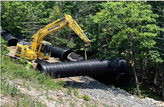
CLH is laying out pipe that will be used to slip line the Dunstan River crossing
