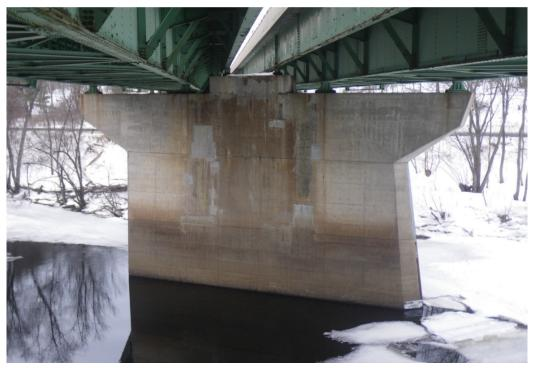
Figure 2 View of Pier Concrete Deficiencies.
