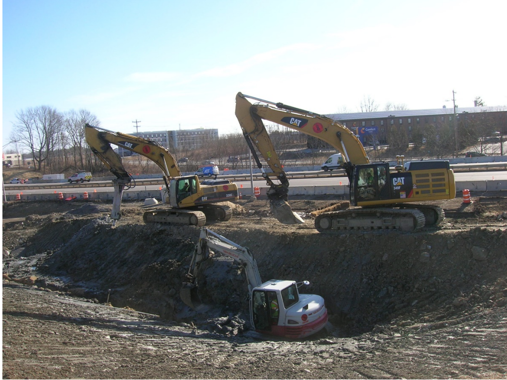
Constructing Underdrain Soil Filter (USF) basin in at mile 45.8.
