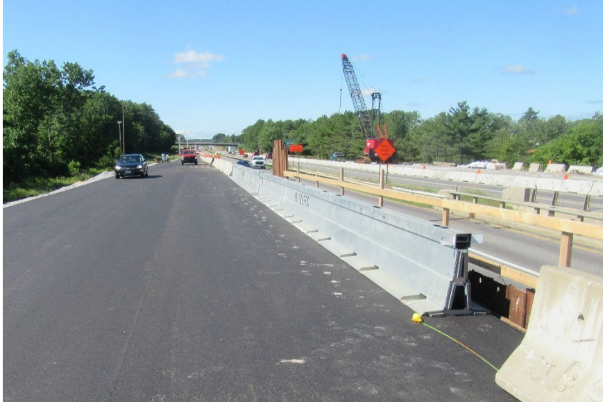
Installing temporary barrier northbound for phase 2
