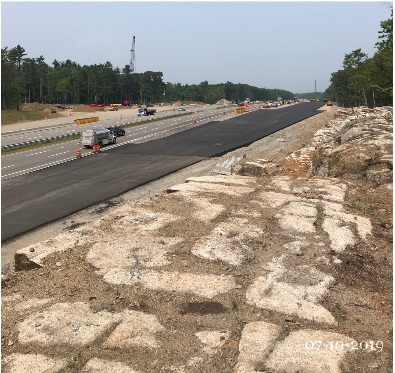
Paving northbound – looking at toll plaza cash lane area
