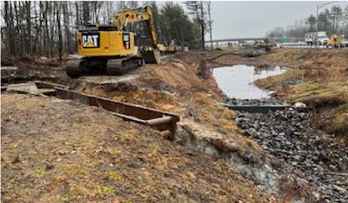
Installation of Drainage at Underground Soil Filter #1 (USF 1).
