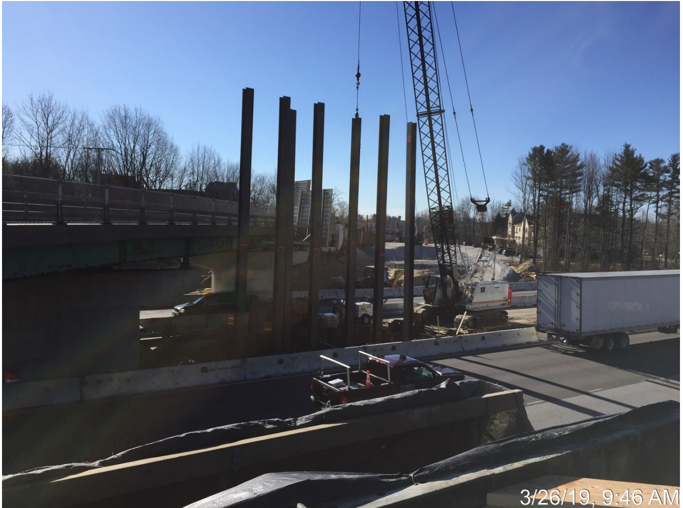
H-pile for pier 1
