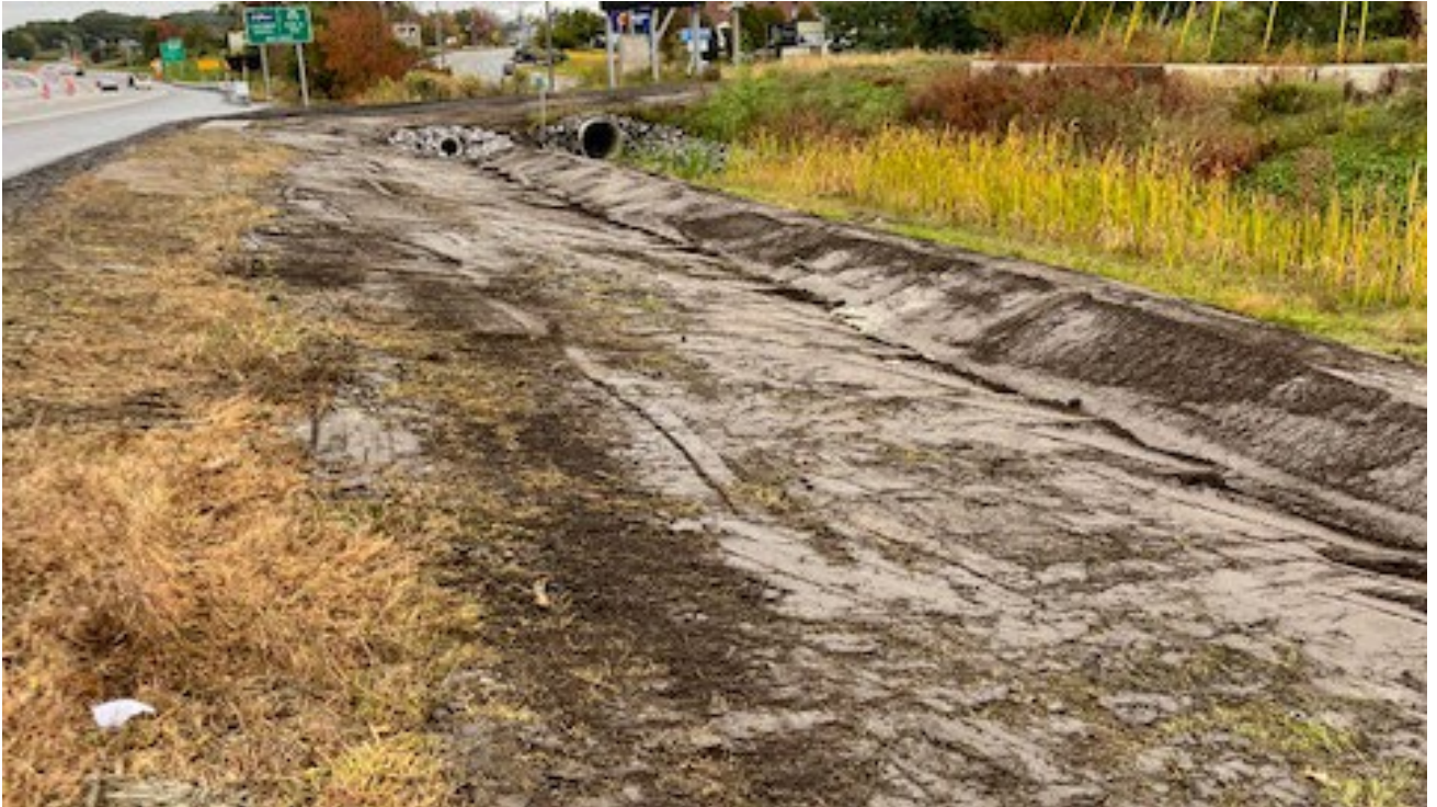
Completed repairs to underdrain soil filters located northbound in South Portland
