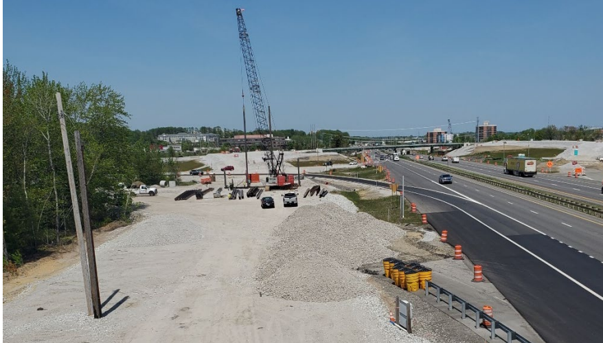
Driving H-pile SB on-ramp new toll plaza
