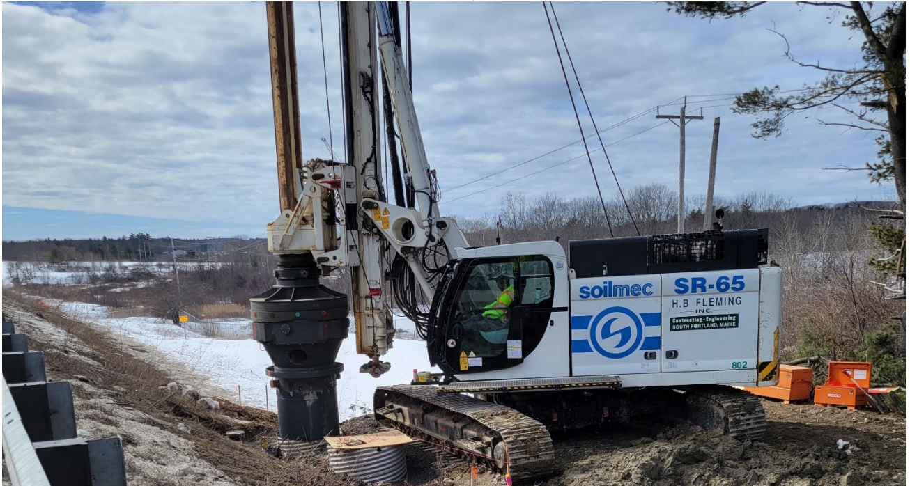
Installation of overhead sign structure foundation
