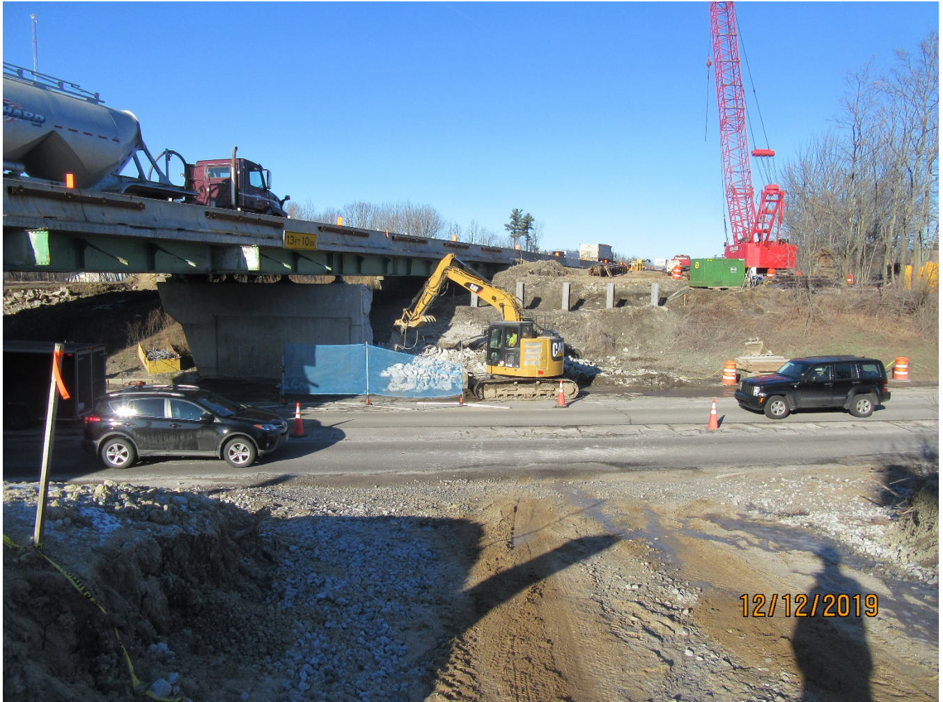
Warren Avenue northbound bridge work
