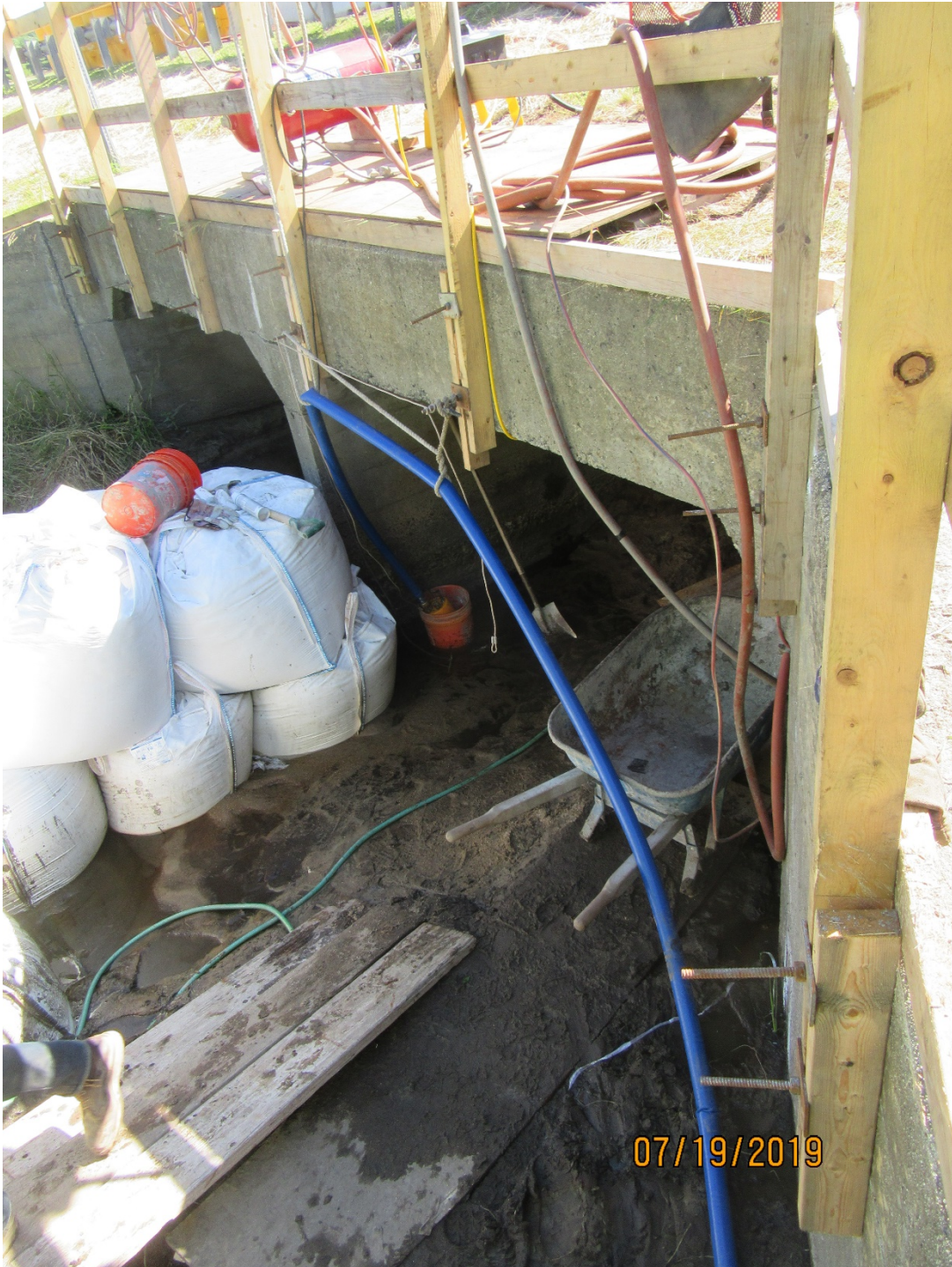
Cole Brook box culvert repair
