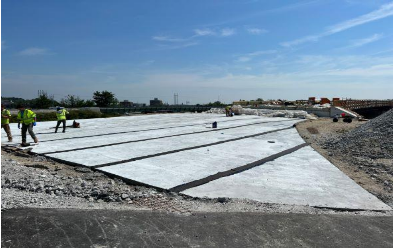
Looking east at crews sealing construction joints on the approach slab
